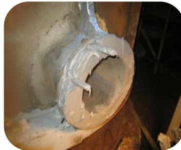
Damaged flange face repaired using 101 Metal Repair Paste
