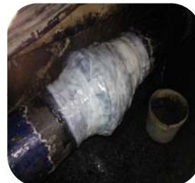
Leaking pipe sockets on a diesel pipeline at a European oil refinery wrapped and sealed using 104 Metal Repair Fluid XF
