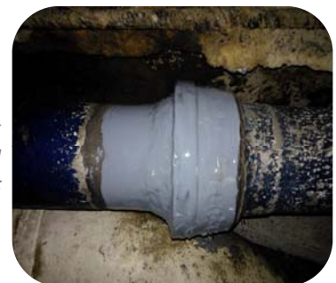
Leaking pipe sockets on a diesel pipeline at a European oil refinery wrapped and sealed using 104 Metal Repair Fluid XF
