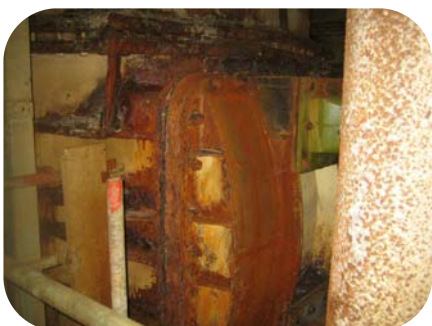
Emergency repair to seal a leaking flange face on a cooler box
