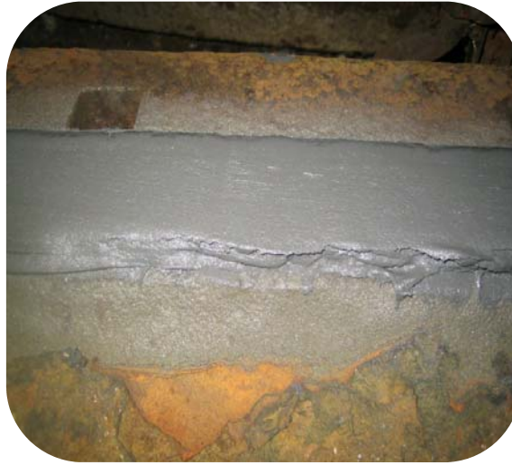
Seal on a process vessel door had been badly corroded from chemical attack. The seal surface was re-formed using 101 Metal Repair Paste
