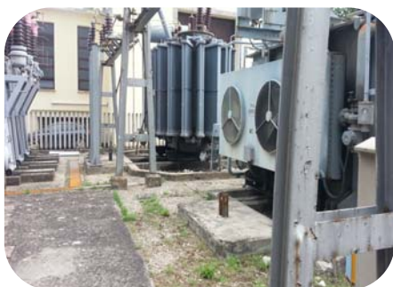
Weeping transformer surfaces manually abraded and sealed using 104 Metal Repair Fluid XF
