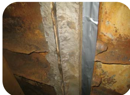
Emergency repair to seal a leaking flange face on a cooler box
