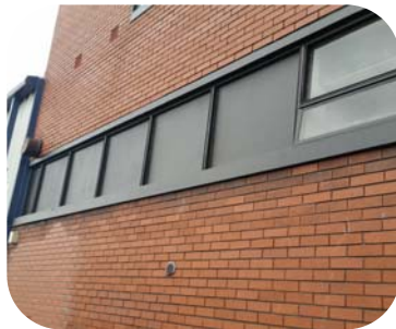
Training facility in the UK was refurbished using Resimac corrosion protection systems. All surfaces were mechanically abraded and primed with 506 Aluprime and top coated with 508 UVPU
