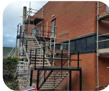
Training facility in the UK was refurbished using Resimac corrosion protection systems. All surfaces were mechanically abraded and primed with 506 Aluprime and top coated with 508 UVPU
