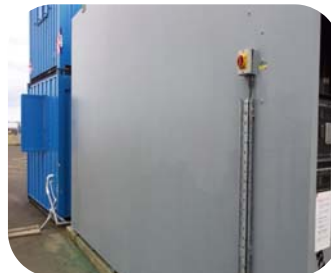
Diesel storage tank at a UK marina was badly corroded due to the corrosive environment. The external tank surfaces were mechanically abraded and protected using Resichem 501 CRSG.
